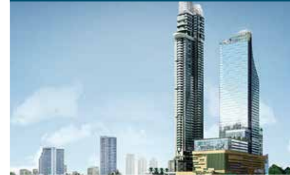
Canapaya Residence Tower
